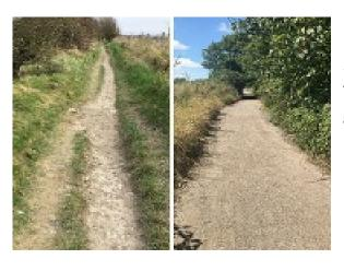
560m length of bridleway was gullied and slippery in the wet due to underlying chalk. The path was regraded and surfaced to provide a wider, level path for users providing a useful off-road link between Lancing College and the South Downs. The works were undertaken in August 2024.
